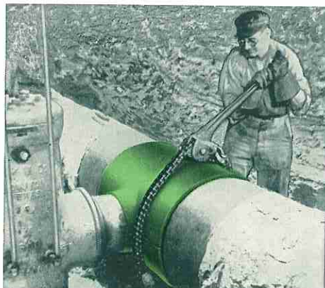
Field photographs showing progressive stages of making branch connection to an in-service line and reinforcing it with the Ladish Split Tee
