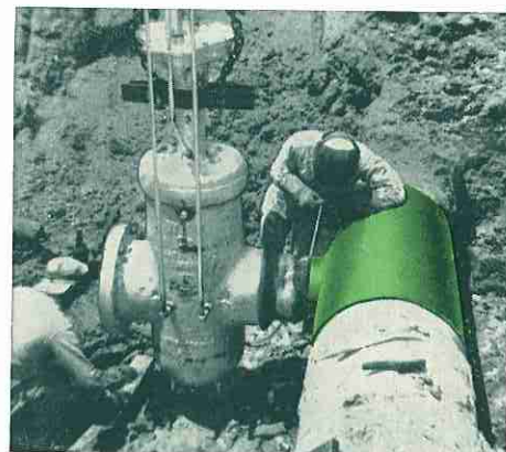
Field photographs showing progressive stages of making branch connection to an in-service line and reinforcing it with the Ladish Split Tee
