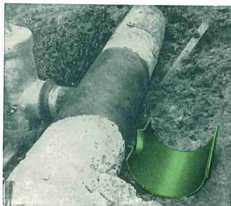
Field photographs showing progressive stages of making branch connection to an in-service line and reinforcing it with the Ladish Split Tee
